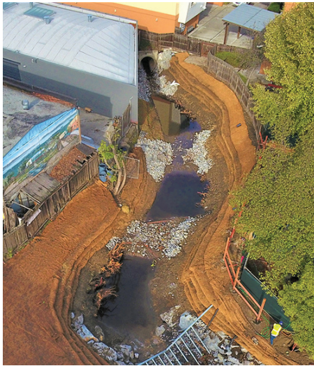
Codornices Creek Restoration Skyview
